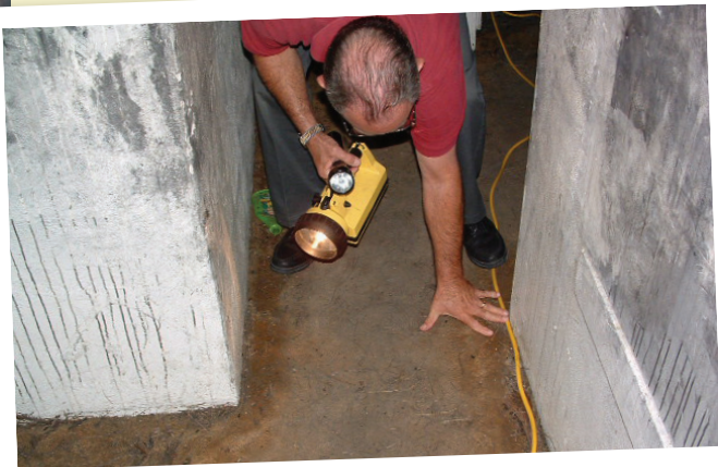
Figure B Two consecutive offset turns and this narrow hallway made it difficult for fire fighters to maneuver.
